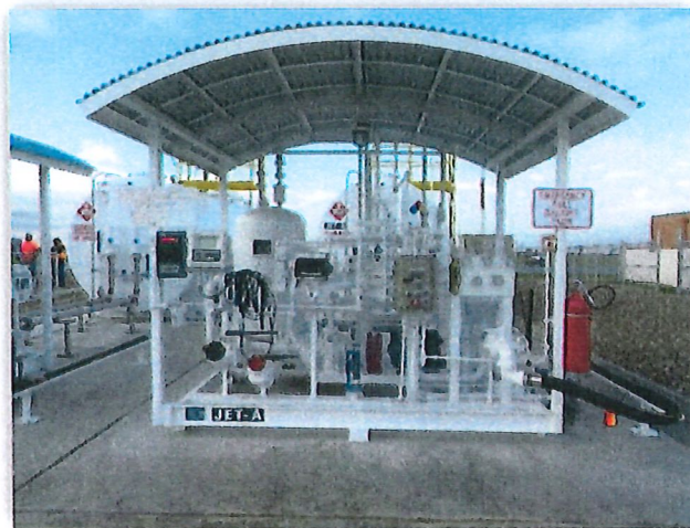
Typical Bulk Loading, Unloading and Recirculation Skid
