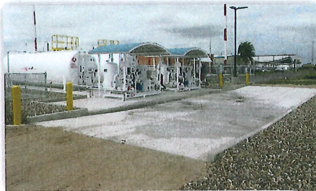
Typical “Drive-In” Truck Containment Pad
